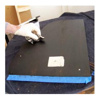
Now that the back crack is glued and closed, I could sand down the area to remove any residual glue and to smooth out a few of the scratches and slight gouges that occurred over the years.
