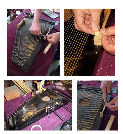
The two blocks that the chord bar top fastens to were cracked and one piece was broken and missing. I used a small chisel to square off the broken piece and glued in a small basswood replacement. At the same time I injected glue into the other cracks, where the screws had pulled out, and clamped them shut.
