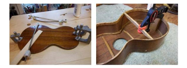
On this day I fixed the back crack. I used special curved violin clamps to pull the sides together to close the crack after applying glue. I also glued and clamped the broken back brace.
